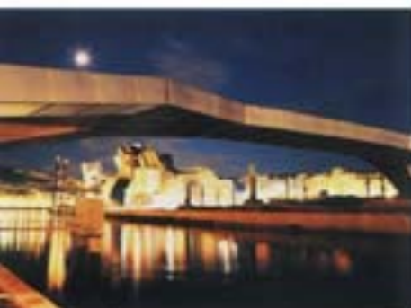
Pasarela peatonal Pedro Arrupe
